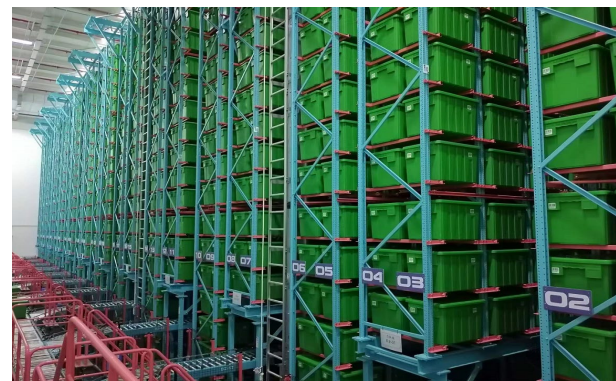
Automatic warehousing equipment
